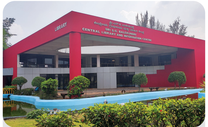
Visvesvaraya Technological University, Belgaum
